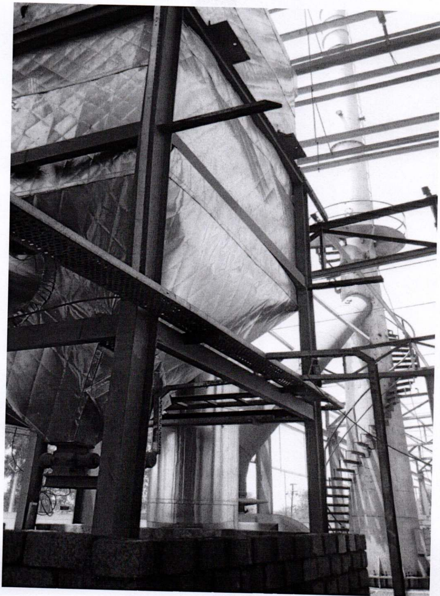
Annexure No. 07 (A) Boiler bag filter housing
