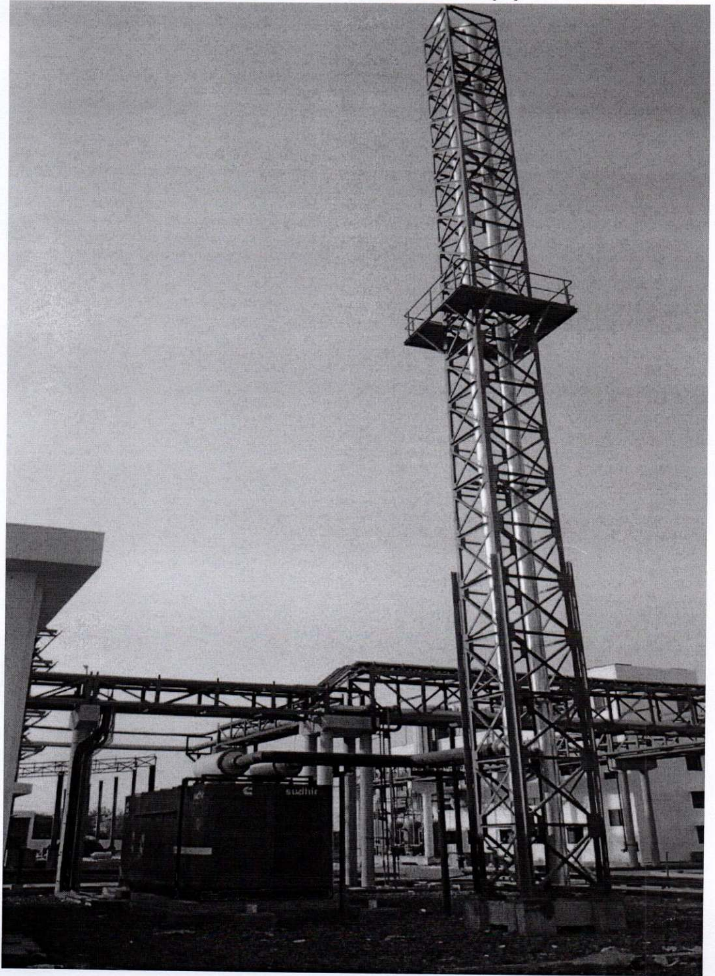
Annexure No. 08 DG Stack (A)
